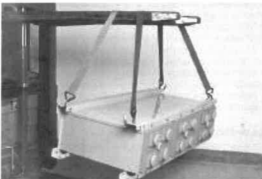
Figure 5: Positioning the module onto the base channels
