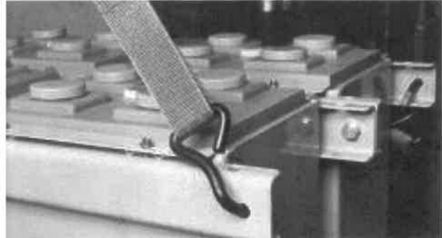
Figure 3: Lifting strap/hook attached to a module
