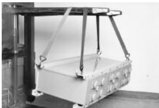
Figure 5: Positioning the module onto the base channels
